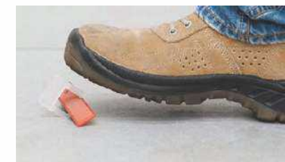
6. Remove Wedges ones it Dry
