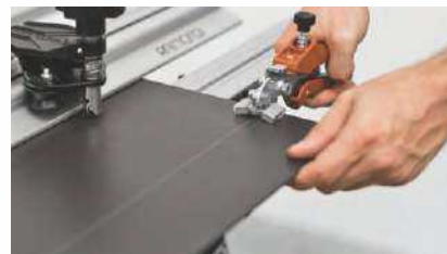
2. Cutting of Tile
