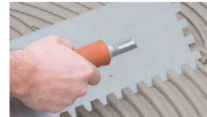
1. Cement laying on Floor
