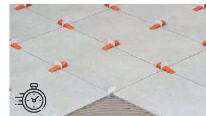
5. After Levelling Process leave it for 8-10 hrs.
