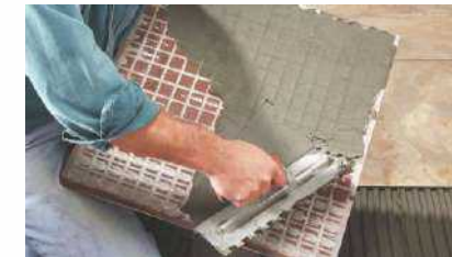
2. Cement laying on Tile
